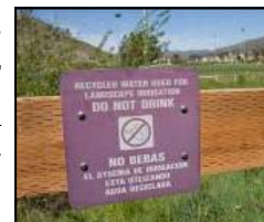
Recycled water is designated by purple pipes and signs
